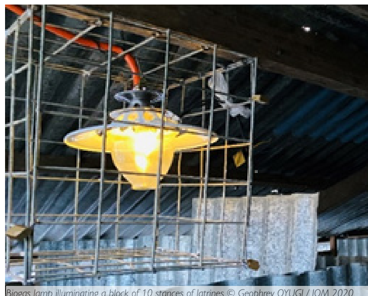
Biogas lamp illuminating a block of 10 stances of latrines © Geophrey OYUGI / IOM 2020
