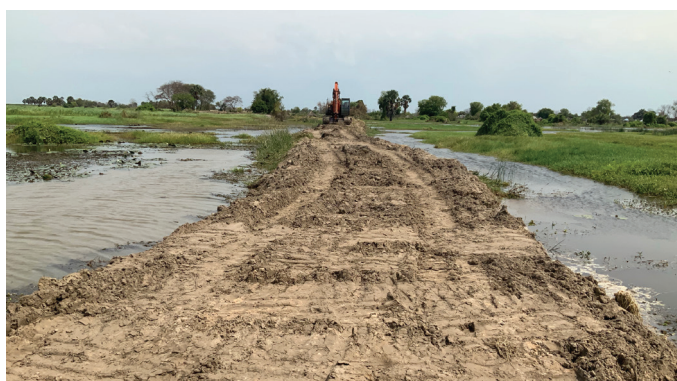
Bor Dike Repair Work ©IOM 2021 / Moses Alier
