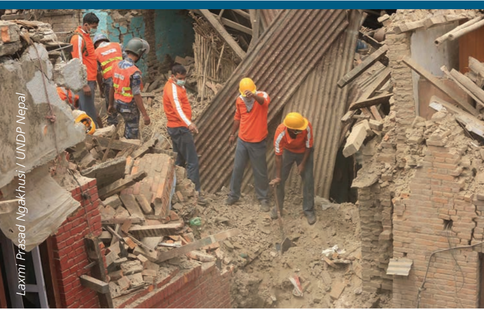
Some of the damage in Bhaktapur.
