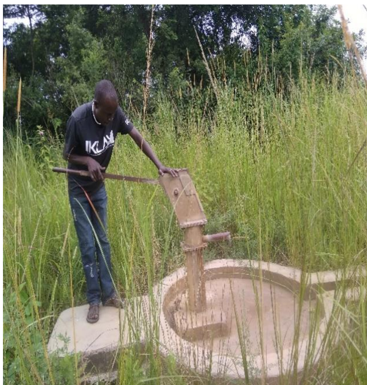
Figure 3: Sera Jale BH which is broken down and needs repair, currently community are collecting drinking water from Nyawa River.
