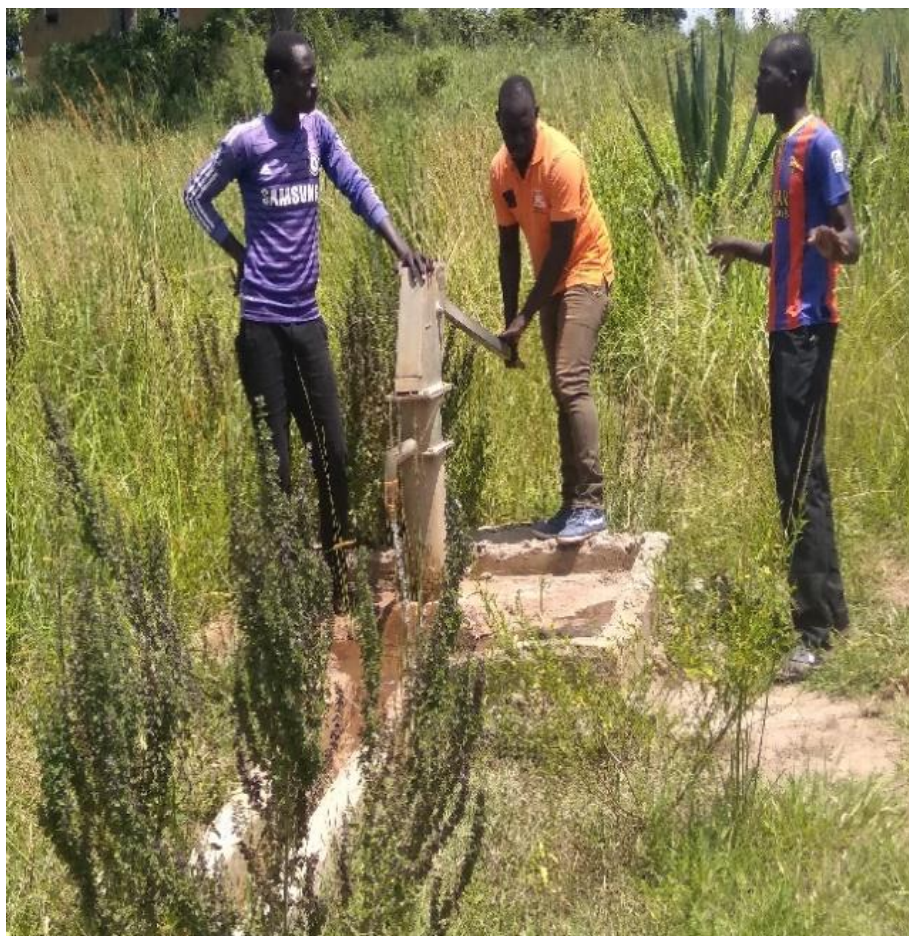
Figure 4: The BH is functional but it has loose pedestal and produces brownish water which not sufficient for human consumption.
